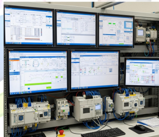
Live Monitoring System
